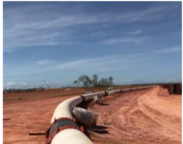
Figure 3. Curved installation of 900 mm ISO Victaulic Style 908 couplings.
