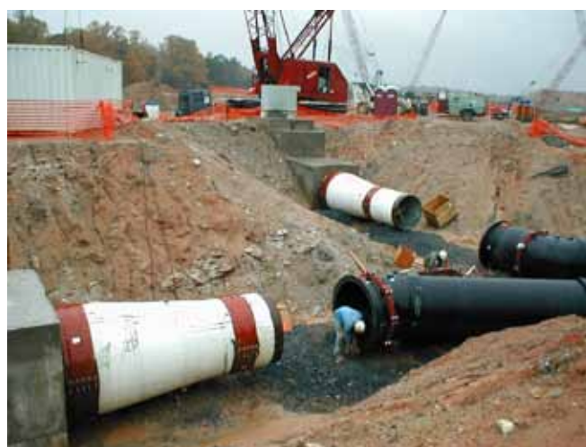
SHOAL CREEK, GA 60 & 72"/1500 & 1800MM VICTAULIC BOLTED SPLIT SLEEVE AND STYLE 44 VIC-RING COUPLINGS
