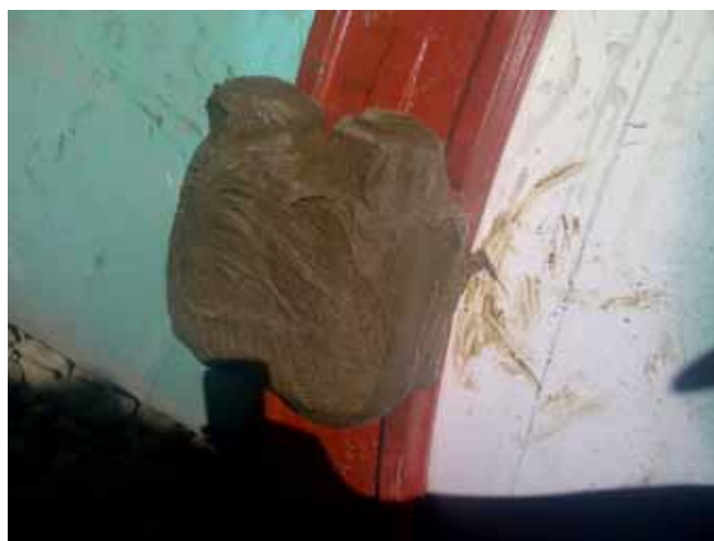
FIELD APPLIED WAX TAPE COVERING BOLTS ON VICTAULIC AGS COUPLING
