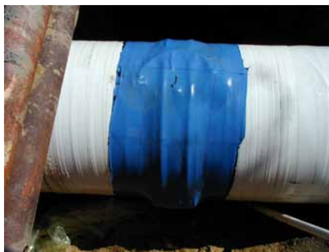
FIELD APPLIED HEAT SHRINK COVERING JOINT
