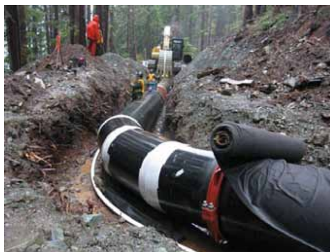
36"/900MM VICTAULIC AGS STYLE W77 FLEXIBLE COUPLINGS DIRECT BURIED PENNSTOCKVANCOUVER ISLAND, BC CANADA
