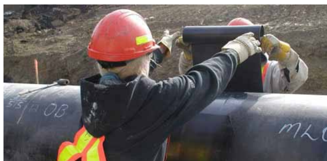
INSTALLATION OF ASPHALTIC TAPE WRAP
