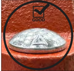
OVAL NECK OF BOLT SEATED PROPERLY
