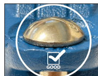
OVAL NECK OF BOLT SEATED PROPERLY
