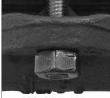
7. INSTALL BOLT AND NUT: Install the bolt into the outlet housing, as shown to the left, and thread a nut onto the bolt. NOTE: Verify that the oval neck of the bolt seats properly in the bolt hole. DO NOT tighten the nut completely. The bolt pads need to be set at a gap for reinstallation of the coupling. The nut should be flush with the top of the bolt to provide the proper gap.
