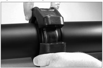
**5. INSTALL HOUSINGS:** Install the housings over the gasket. Make sure the housings' keys engage the grooves properly on both pipe/fitting
