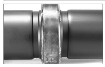
**4. JOIN PIPE/FITTING ENDS:** Align and bring the two pipe/fitting ends together. Slide the gasket into position and center it between the groove in each pipe/fitting end. Make sure no portion of the gasket extends into the groove in either pipe/fitting end.
