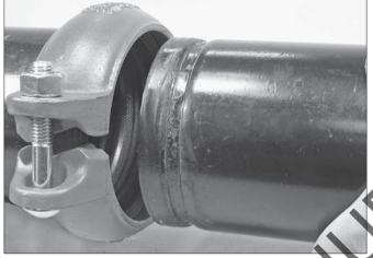
**5. ASSEMBLE JOINT:** Assemble the joint by inserting the groeved and of a pipe/mating component into each opening of the coupling. The ends of the grooved pipe/mating components must be inserted into the coupling until contact with the center leg of the gasket occurs. A visual check is required to ensure the coupling keys align with the grooves in the pipe/mating components. **NOTE:** The coupling may be rotated to ensure the gasket is seated properly.
