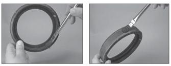
3. FOR RE-INSTALLATION OF STYLE 177 COUPLINGS, LUBRICATE GASKET: Apply a thin coat of Victaulic Lubricant or silicone lubricant to the gasket sealing lips and exterior. It is normal for the gasket surface to have a hazy white appearance after it has been in service.
