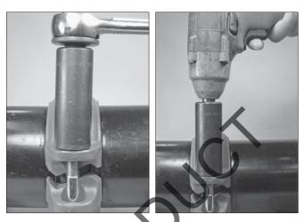
**6. TIGHTEN NUTS:** Tighten the puts evenly by alternating sides until metal-to-metal contact occurs at the bolt pads. The middle section of the bolt pad mating surfaces must be in full metal-to-metal contact to ensure a properly assembled joint. Make sure the housings' keys engage the grooves completely during tightening.
