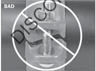
7. Visually inspect the bolt pads at each joint to ensure metal-to-metal contact is achieved across the entire bolt pad section.
