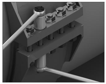
10. Finish closing the coupling bodies by tightening each set of hardware gradually, alternating between the two closure plate locations, until the coupling bodies are in full contact with the pipe around its circumference. The closure plates should not contact each other.
