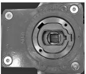
3. Turn the handwheel counterclockwise. Verify that the valve is in the fully "open" position by checking the position indicator on top of the stem, as shown to the left. The position indicator line on top of the stem should be perpendicular to the "shut" position.
