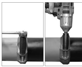
**6. TIGHTEN NUTS:** Tighten nuts evenly by alternating sides until metalto-metal contact occurs at the bolt pads. Verify that the oval neck of each bolt seats properly in the bolt hole and that housings' keys engage the grooves completely on both mating components.
