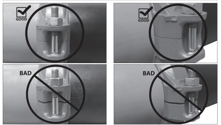
7. Visually inspect the bolt pads at each joint to verify that metal-to-metal contact is achieved across the entire bolt pad section.
