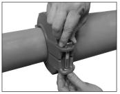
**6. INSTALL BOLTS/NUTS:** Install the bolts and thread a nut fingertight onto each bolt. **NOTE:** Verify that the oval neck of each bolt seats properly in the bolt hole.
