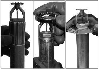
2. Carefully place the sleeve, recessed collar, or flush plate over the sprinkler and onto the barrel.
