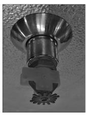
3. Reinstall the bulb protector onto the sprinkler until the sprinkler system is placed in service. Use caution when reinstalling the bulb protector to prevent damage to the bulb, deflector, and frame arms. DO NOT use any tools to reinstall the bulb protector.
