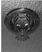
2. Install the skirt or recessed escutcheon. Verify that the skirt or recessed escutcheon is in full contact with the freezer ceiling or wall, as shown above.
