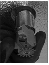
1. After the dry sprinkler has been installed properly, in accordance with the I-40 Victaulic® FireLock™ Automatic Sprinklers Installation and Maintenance Instructions, temporarily remove the bulb protector from the sprinkler. Use caution when removing the bulb protector to prevent damage to the bulb, deflector, and frame arms. DO NOT use any tools to remove the bulb protector.
