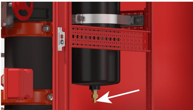
Bleed the valve, located at the bottom of the air tank, once every three months to remove any moisture from the line.
