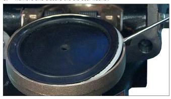
6. Pry the old clapper seal out of the clapper. For 1½ – 3-inch/DN40 – DN80 and 8-inch/DN200 sizes, verify that the seal ring is removed with the clapper seal. Discard the old clapper seal and replace it with a new, Victaulic-supplied clapper seal assembly. Proceed to step 6a for 1½ – 3-inch/DN40 – DN80 and 8-inch/DN200 sizes or step 7 for all other sizes.
