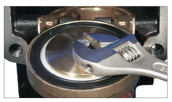
11. Install the seal assembly bolt/bolt seal through the seal retaining ring and clapper. Tighten the seal assembly bolt/bolt seal to the torque value listed in the table below to ensure a proper seal.
