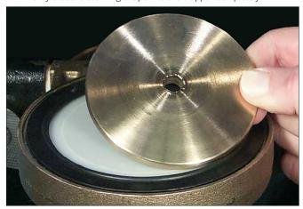
Place the seal retaining ring (flat side down) onto the seal washer of the clapper seal, as shown above.
