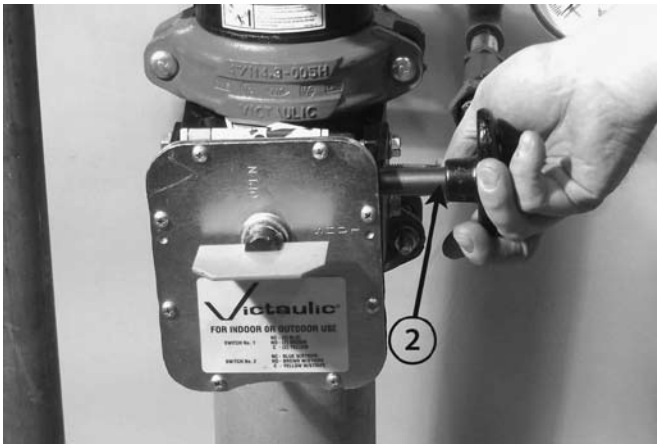
7. Close the water supply main control valve (2).
