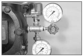
**2.** Remove the valve from service. Make sure there is "zero" pressure on all gauges.
