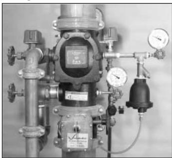
${\bf 6.}$  Insert the tubing from the Series 75D Water Column Kit into the drip cup, located at the back of the valve.
