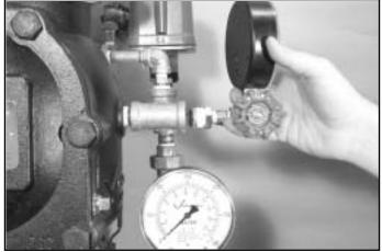
**3.** Remove the reducing bushing/nipple/gauge valve assembly from the tee on the system side of the dry or actuated check valve.
