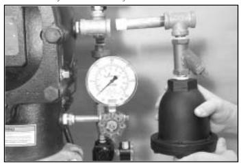
${f 4.}$  Install the Series 75D Water Column Kit into the tee where the gauge valve assembly was removed in step 3.
