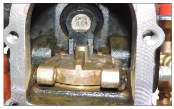
**5.** Place the new clapper assembly onto the valve body seat ring. Ensure that the holes in the clapper arms align with the holes in the valve body.
