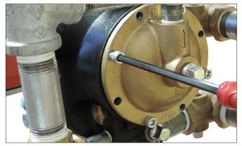
**3.** Remove the cap screws from the diaphragm cover, and pull the diaphragm cover/trim off the valve.
