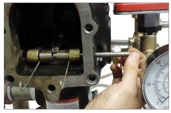
**3.** Remove the clapper shaft. **NOTE:** As the shaft is being removed, the clapper spring will drop out of position. Save the clapper spring for re-installation.
