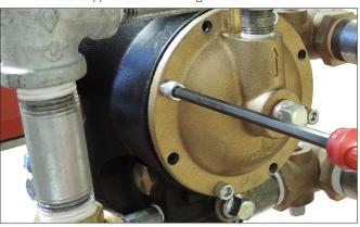
**3.** Remove the cap screws from the diaphragm cover, and pull the diaphragm cover/trim off the valve.
