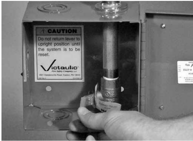
19. Open the manual pull station to bleed off any air that is present.
