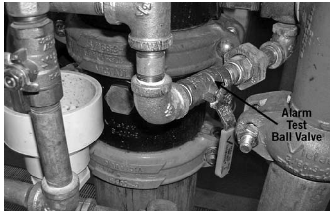
10. Confirm that the alarm test ball valve is closed.
