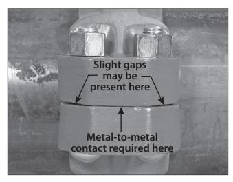
11. INSPECT BOLT PADS: Before pressurizing the system, inspect the bolt pads at each joint to ensure proper assembly is achieved.
