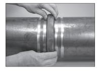
4b. POSITION ENDSEAL<sup>TM</sup> GASKET: Insert the grooved pipe end into the gasket until it contacts the center leg of the gasket.
