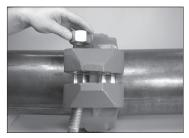
9. INSTALL BOLTS AND NUTS: Install the bolts, and thread a nut finger-tight onto each bolt. Verify that the oval neck of each bolt seats properly in the bolt hole.
