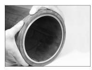
**4a. POSITION STANDARD GASKET:** Position the gasket over the pipe end. Verify that the gasket does not overhang the pipe end to prevent pinching, cutting, or rolling the gasket.
