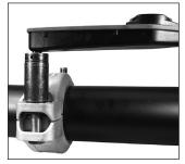
**9. TIGHTEN NUTS:** Tighten the nuts evenly by alternating sides to prevent seal assembly damage (extra-deep sockets are required). Verify that the housings' keys engage the grooves completely on both mating component ends. Apply torque to each nut with a torque wrench. Refer to the markings on the housings or the table on this page for the torque requirement. **NOTE:** It is important to tighten the nuts evenly to prevent pinching of the seal assembly and to achieve even gaps at the bolt pads.
