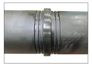
**3b. CENTER GASKET:** Align and bring the pipe ends together. Slide the gasket into position by centering it between the grooves in each pipe end.
