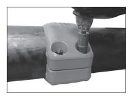
**5b. TIGHTEN NUTS:** Tighten the nuts evenly by alternating sides until metal-to-metal contact occurs at the bolt pads.
