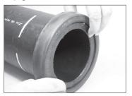
**4. INSTALL GASKET:** Install the gasket over the HDPE pipe end. Ensure that the gasket does not overhang the pipe end.
