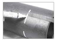
2. MARK PIPE FOR GASKET: Refer to the "Pipe Insertion Depth" column in the table on page 31. Using a measuring tape and a brightly-colored pencil or paint stick, mark the HDPE pipe end at the measurement listed in this table. This mark will be used for visual inspection to ensure that the pipe is inserted properly in the coupling. Make at least four marks, equally spaced around the circumference of the pipe ends.
