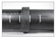
**6. ALIGN GASKET:** Align and bring the pipe ends together. Slide the gasket into position by centering it between the first set of pipe marks. **NOTE:** The space between the pipe ends must never exceed ½ inch/6 mm for 2–4-inch/50–100-mm sizes and ½ inch/8 mm for 5-inch/125-mm and larger sizes.
