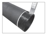
**4. LUBRICATE PIPE ENDS:** Apply a thin coat of lubricant to the HDPE pipe end, from the end of the pipe to the paint mark made in step 3.
