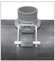
**9. POSITION FOR TIGHTENING:** Position the U-bolts, crossbars, and strap so that a deep well socket can fit around all nuts for tightening.
