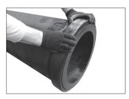
**3a. POSITION GASKET:** Position the gasket over one pipe end. Verify that the gasket does not overhang the pipe end.
