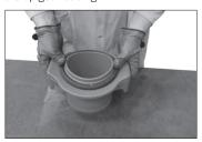
**5. INSTALL O-RING:** Press the o-ring into the groove on the underside of the spigot housing. Do NOT place the o-ring on the pipe and then attempt to push the locating collar through it. This may push the o-ring into the hole, and will prevent proper sealing.
