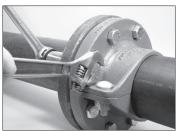
11. TIGHTEN NUTS: Tighten all nuts evenly in a crossing pattern, in accordance with a regular flange assembly. Continue to tighten all nuts until the standard, flanged joint torque requirement is reached.
