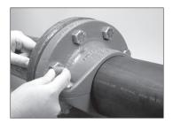
10. INSTALL BOLTS: Join the mating flange with the flange adapter by aligning the two bolts with the mating flange holes. Install the remaining standard bolts through the flange adapter and mating flange. Thread a nut onto the end of each bolt.
