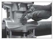
**5c. REMOVE ONLY THE SPACER BOLTS:** There is one spacer bolt on each bolt pad to maintain spacing between the bolt pads during shipping and assembly. After inserting pipes, remove only the spacer bolts and the attached warning tags before tightening the four nuts in step 6.
