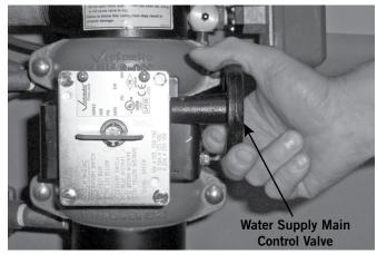
4. Close the water supply main control valve to take the system out of service.
