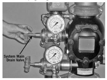
8. Open the system main drain valve to drain any water that has accumulated and to release system air pressure.
