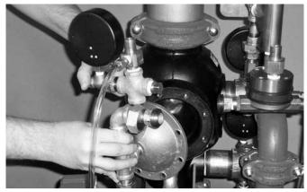
2. Remove the cap screws from the diaphragm cover, and pull the diaphragm cover/trim off the valve.
