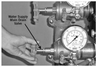
2. Open the water supply main drain valve fully to flush the water supply of any contaminants.
