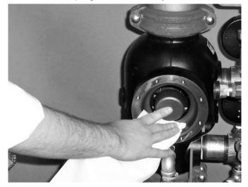
4. Clean the back of the valve body to remove any debris that may interfere with proper diaphragm seating.
