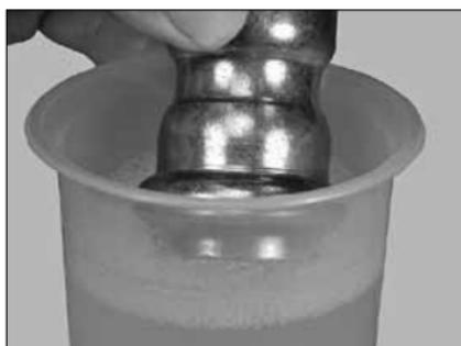
**SI LE PRODUIT REÇU N'EST PAS DANS UN SAC D'EMBALLAGE DE L'USINE, SES JOINTS D'ÉTANCHÉITÉ NE SONT PAS PRÉ-LUBRIFIÉS ET DOIVENT ÊTRE LUBRIFIÉS DE LA FAÇON SUIVANTE :**
