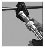
**4.** Make sure the pipe marks indicate full insertion into the coupling or fitting before performing the pressing operation.
