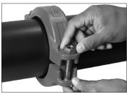
**6. INSTALL BOLTS/NUTS:** Install the bolts, and thread a nut finger-tight onto each bolt. **NOTE:** Verify that the oval neck of each bolt seats properly in the bolt hole.
