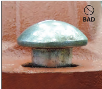
BAD BOLT ENGAGEMENT (OVAL NECK OF BOLT IS NOT SEATED PROPERLY IN THE BOLT HOLE)
