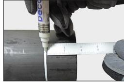
**3. MARK PIPE:** Using a ruler, measuring tape, or the cardboard sleeve and a paint stick, place a mark from the HDPE pipe end around the full circumference:
