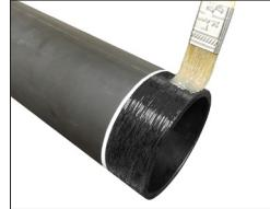
**4. LUBRICATE PIPE END:** Apply a thin coat of lubricant from the end of the pipe to the paint mark made in step 3.
