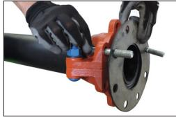
**8. INSTALL FLANGE BOLTS AND NUTS:** Insert lubricated flange bolts through the flange bolt holes and flange gasket (when applicable). Join the mating flange with the flange adapter by aligning the bolts with the mating flange holes. Thread nuts finger-tight onto each bolt. **NOTE:** Flange bolts, nuts, and flange gasket are not provided.
