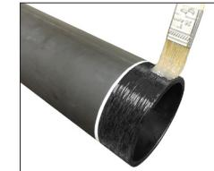
**5. LUBRICATE PIPE END:** Apply a thin coat of lubricant to the pipe end, from the end of the pipe to the paint mark made in step 4.
