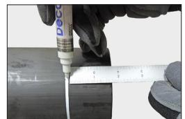
**4. MARK PIPE:** Using a ruler, measuring tape, or the cardboard sleeve and a paint stick, place a mark from each HDPE pipe end around the full circumference:
