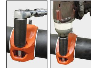
**7. TIGHTEN NUTS:** Tighten the nuts evenly by alternating sides until metal-to-metal contact occurs at the bolt pads. Larger coupling sizes with four bolts shall be tightened in a crossing pattern, as shown. Ensure that the oval neck of each bolt seats properly in the bolt hole.
