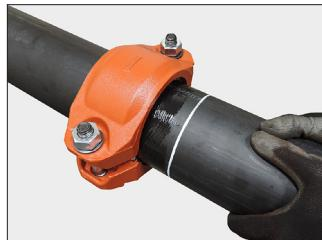
**6b.** Bring the second HDPE pipe end to meet the first HDPE pipe end, then slide the coupling back until evenly spaced between the pipe insertion marks.
