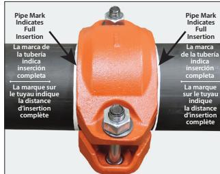
**6c.** The distance from the edge of the coupling housings to the pipe insertion marks must not exceed  $\frac{3}{16}$  inch/5 mm at any point around the circumference of the pipe ends.
