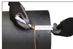
**3. MARK PIPE:** For the HDPE side, use a ruler, measuring tape, or the cardboard sleeve and a paint stick to place a mark from the end of the HDPE pipe around the full circumference:
