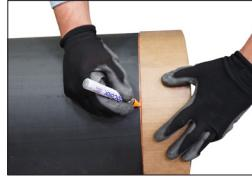
This mark will be used for visual inspection to ensure that the HDPE pipe is inserted properly in the coupling. If a full circumferential mark cannot be achieved, make at least four marks, equally-spaced around the circumference of the HDPE pipe end.
