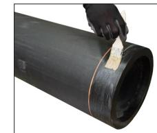
**4. LUBRICATE PIPE ENDS:** Apply a thin coat of lubricant to the HDPE pipe end, from the end of the pipe to the paint mark made in step 3 (as shown in the photo at left). Apply a thin coat of lubricant to the steel mating component end, from the end of the component to the front edge of the groove (as shown by the gray lines in the cross-section diagram below).
