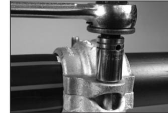
9. Tighten all nuts evenly by alternating sides until metal-to-metal contact occurs at the bolt pads. **NOTE:** It is important to tighten all nuts evenly to prevent gasket pinching.
