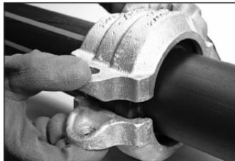
7. Wear gloves while handling coupling housings. The teeth machined into the housings are sharp and can cause injury. Install the housings, making sure the teeth are facing toward the HDPE pipe. The key section of the housings must engage with the shouldered steel pipe end. Make sure the gasket remains positioned properly and that the mark on the HDPE pipe indicates full insertion into the coupling.
