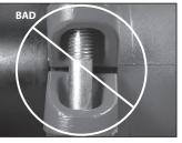
**8.** Visually inspect the bolt pads at each joint to ensure metal-to-metal contact is achieved.
