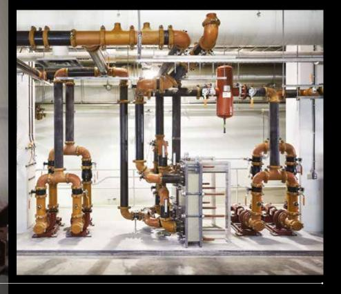
Series 392 Strainer Vibration Isolation Pump Drop
