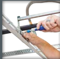
Tighten bracket to ceiling grid
