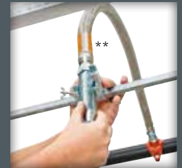
Position sprinkler in bracket
