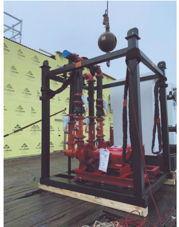
Victaulic components preassembled to a pump and delivered on a skid as a module to lift into place.
