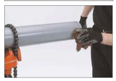
**10.** After the pipe is grooved and the tool is removed, carefully clean chips from the groove with a soft cloth or compressed air.
