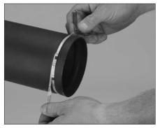
**8.** Carefully check the groove diameter of the pipe ("C" dimension) with the provided Go/No-Go Groove Diameter Tape.
