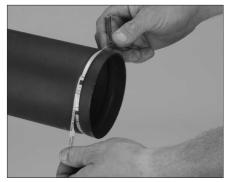
**6.** Carefully check the groove diameter of the pipe ("C" dimension) with the provided Go/No-Go Groove Diameter Tape.
