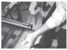
**5.** After a trial groove is prepared and the tool is removed from the pipe, carefully check the groove diameter ("C" dimension), as charted in the "Roll Groove Specifications" section. The "C" dimension is best checked with a pi-tape. It also may be checked with a vernier caliper or narrow land micrometer at two locations, 90° apart, around the groove. The average reading must equal the required groove diameter specification.
