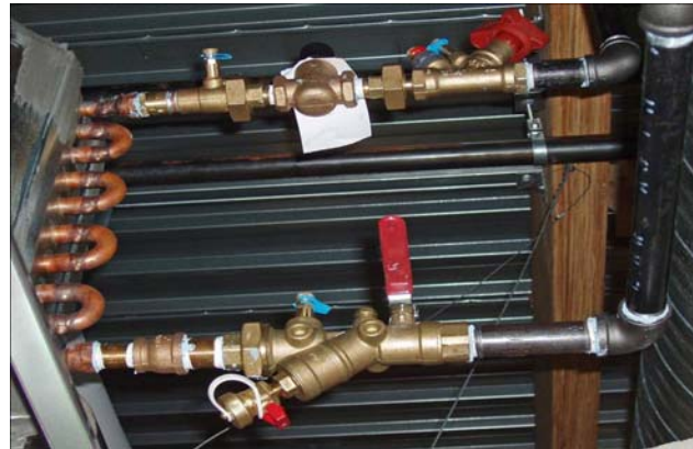
Figure 1: Coil-CW/HW schematic drawing and Tour & Andersson Coil Component
