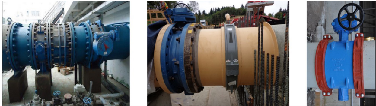
Figure 6. An Example of a Conventional Flanged Valve Assembly (left), an AGS Grooved Coupling (center), and a Grooved Butterfly Valve and AGS Couplings (right)
