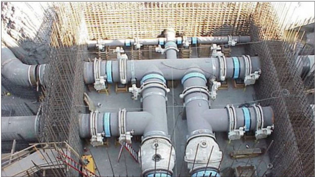
Figure 5. Hydraulic Structure Walls (Thrust taken by walls)
