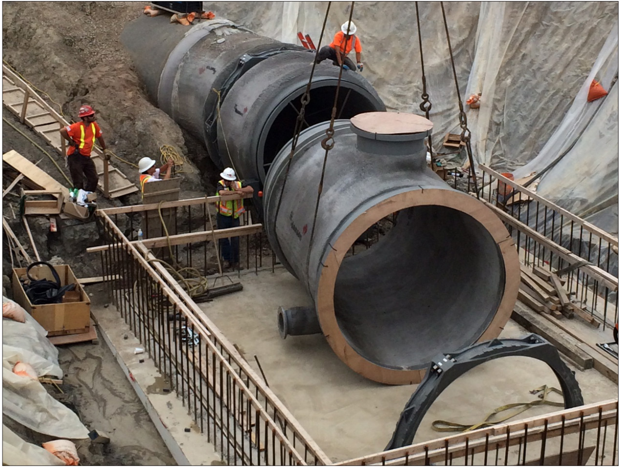
Figure 4. Hydraulic Structure Walls (Thrust taken by grooved flexible couplings)
