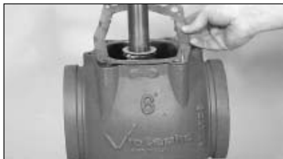
10. Place a new graphite gasket into position.
