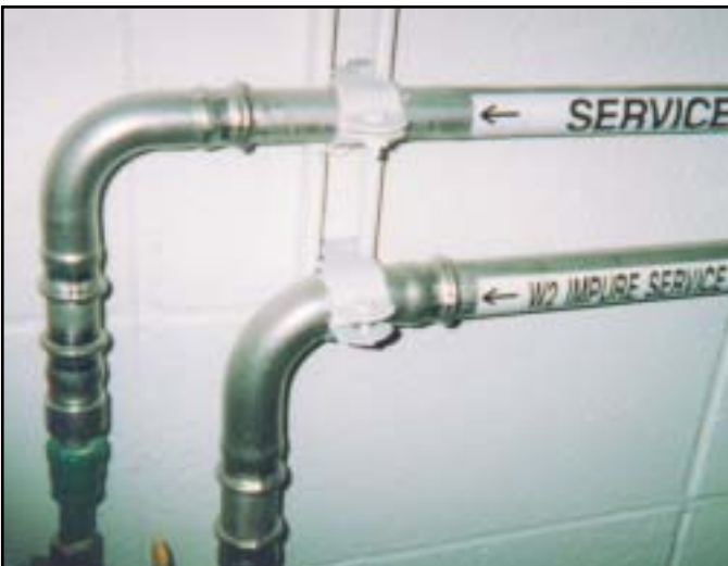
The Pressfit stainless system is ideal for air and water lines. The leak-free joint can be used on systems with pressures up to 300 psi.
