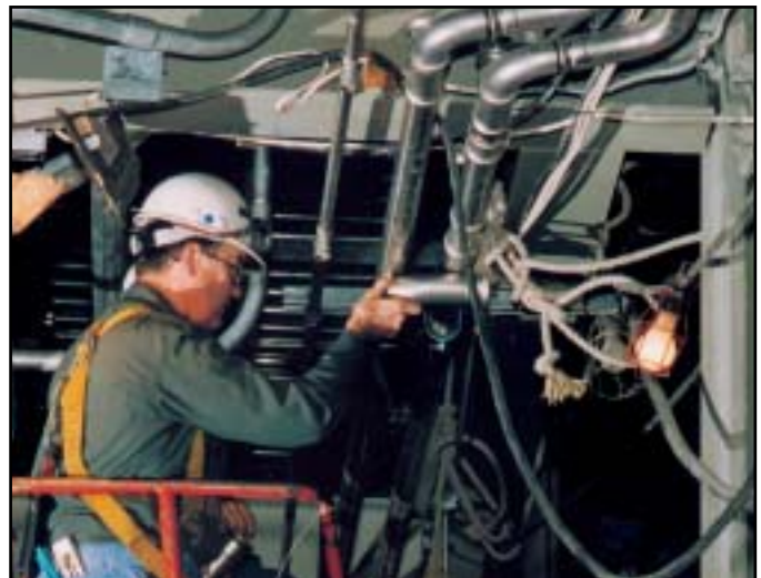
Pressfit products are light in weight, allowing sections to be built on the ground, then joined to the system "in the air." A variety of Pressfit tools are offered to meet the most demanding job site requirements.
